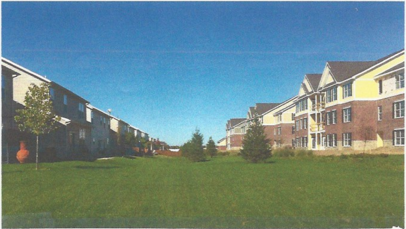
BRIGHTON KNOLL ADJACENT TO APARTMENTS
