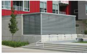
LOUVERED MECHANICAL SCREENS
