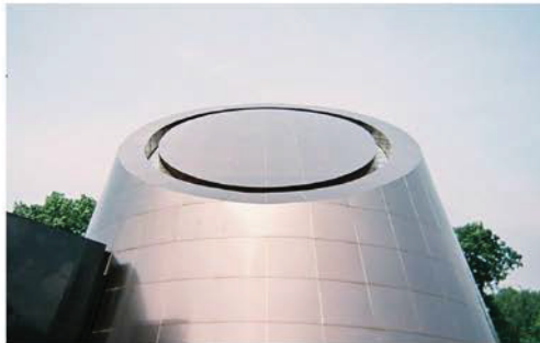
METAL PANEL ROOFS AND FACADE
