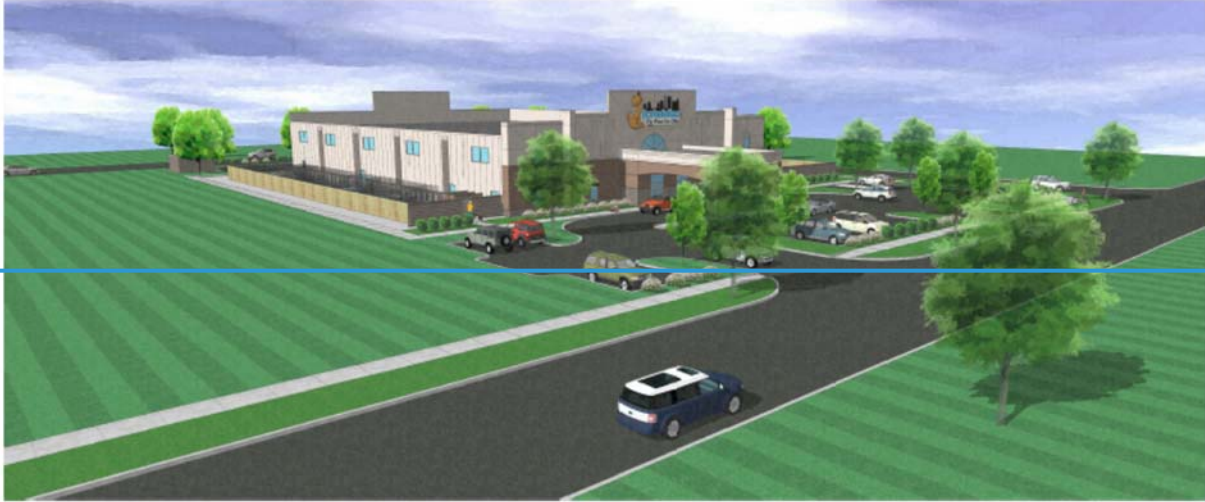
VIEW LOOKING NORTH EAST
