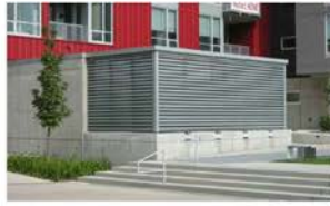
LOUVERED MECHANICAL SCREENS
