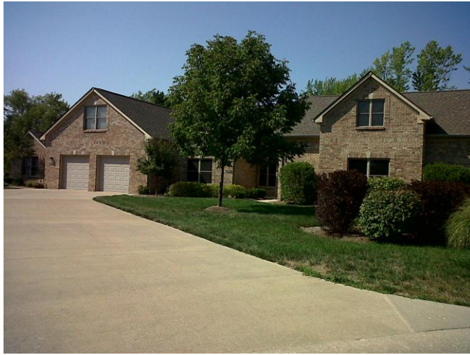
Building Exterior ( see Exhibit 5 in proposed PUD )
