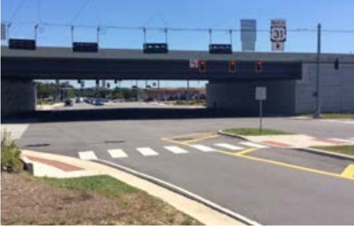
Image 3.1: 151st Street underpass at US Highway 31
