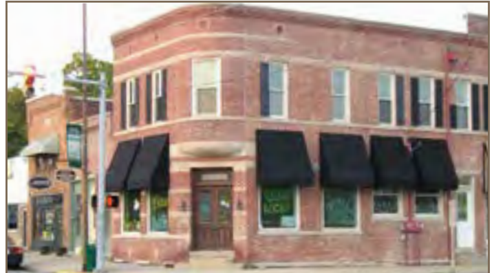
(12) State Bank of Westfield (Contributing), 100 N Union Street. Commercial Vernacular, 1899; Vernacular/Construction (Interim Report No. 022).
