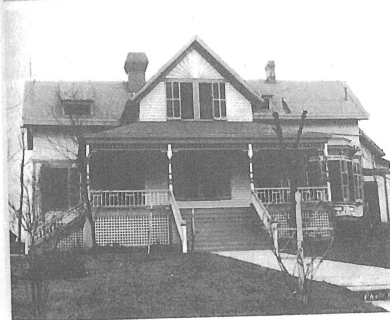
Figure 505 – Side-gabled Roof, One-Story Folk Victorian Examples
