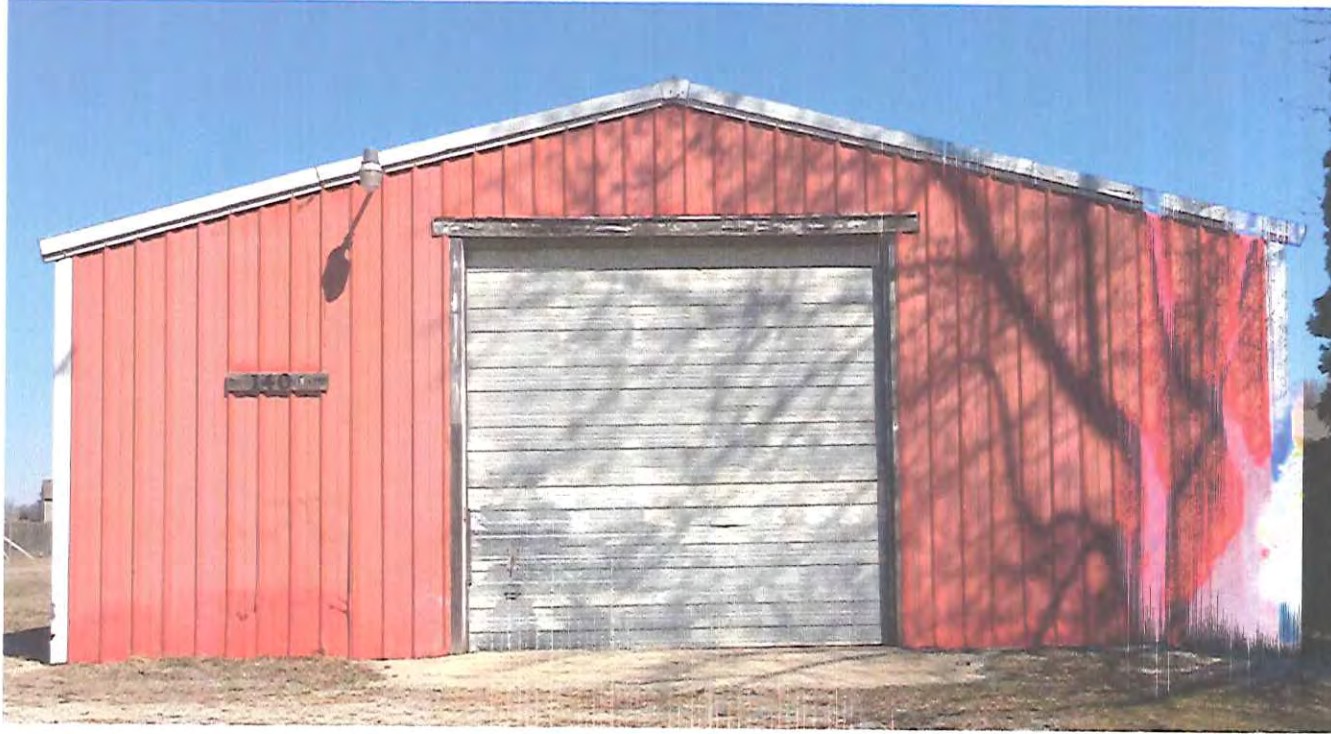
Existing Building (South Side View)
