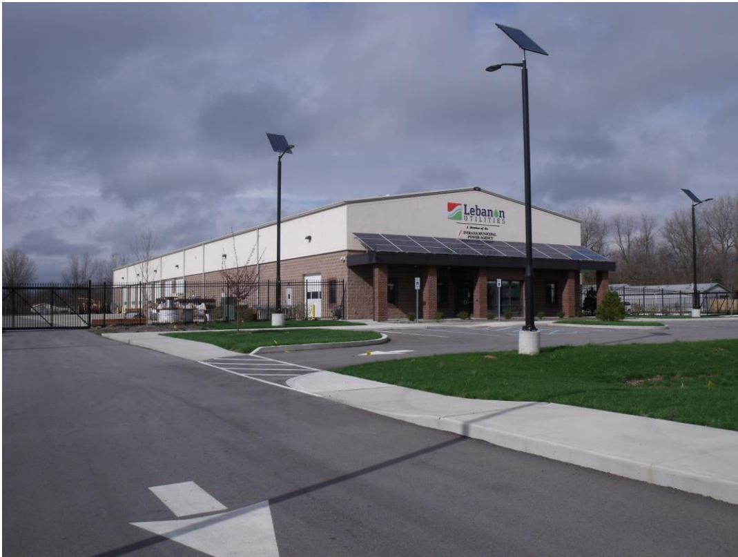
PUBLIC UTILITY – OUTDOOR STORAGE
