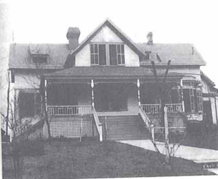
Figure 505 – Side-gabled Roof, One-Story Folk Victorian Examples
