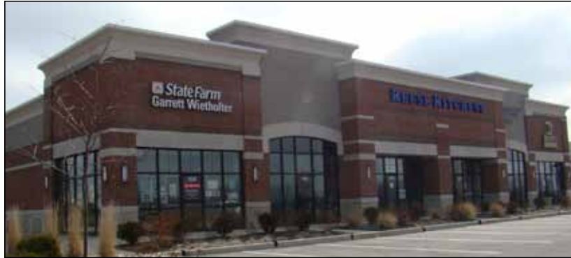
FIGURE 5.3(11): FLAT ROOF - ROOF LINE MODULATION
