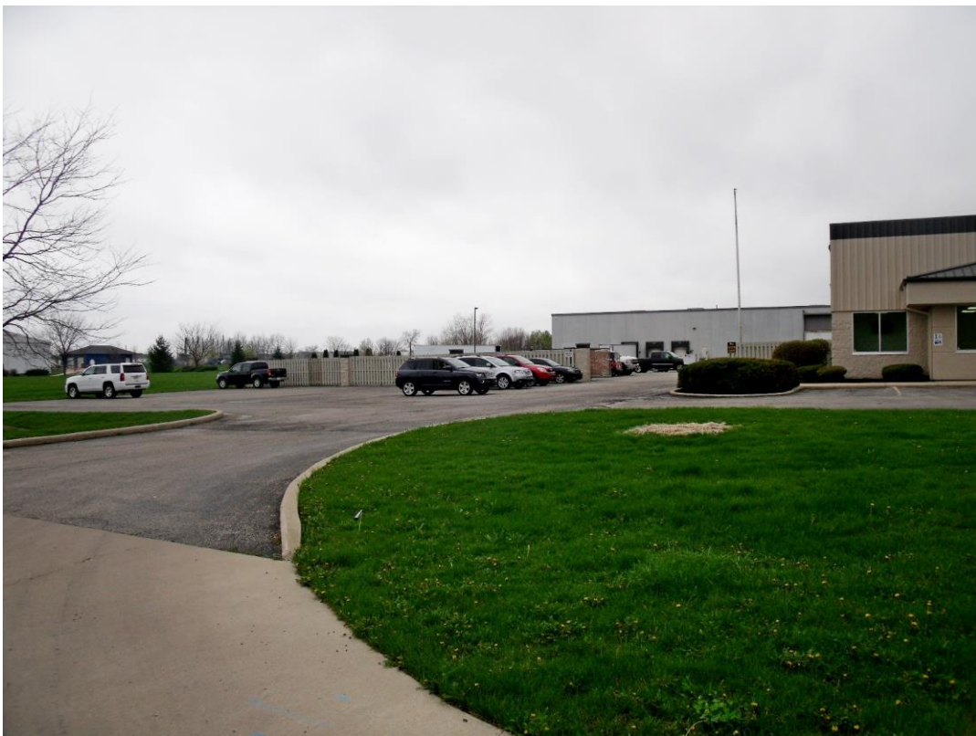
BODY SHOP – SCREENED OUTDOOR STORAGE
