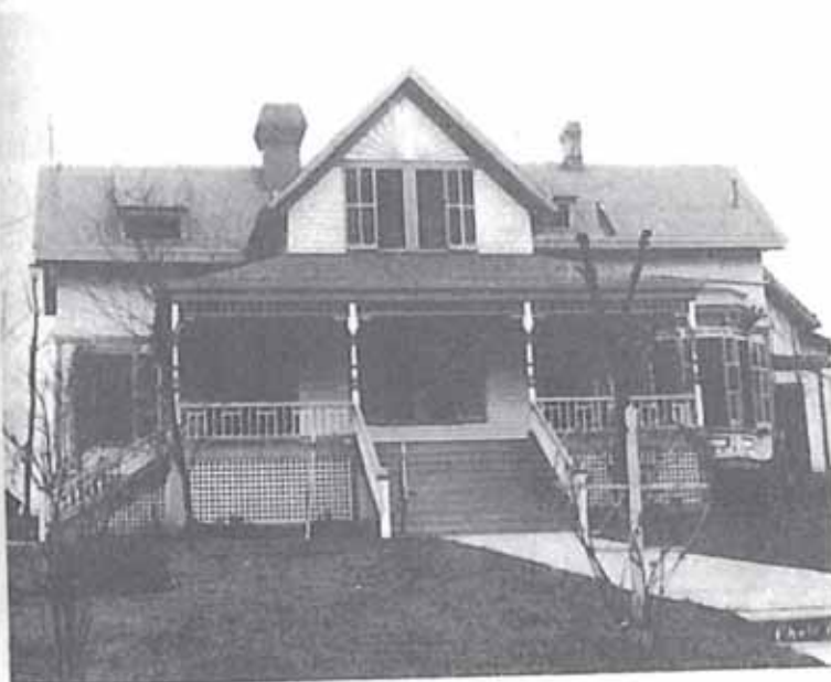
Figure 505 – Side-gabled Roof, One-Story Folk Victorian Examples
