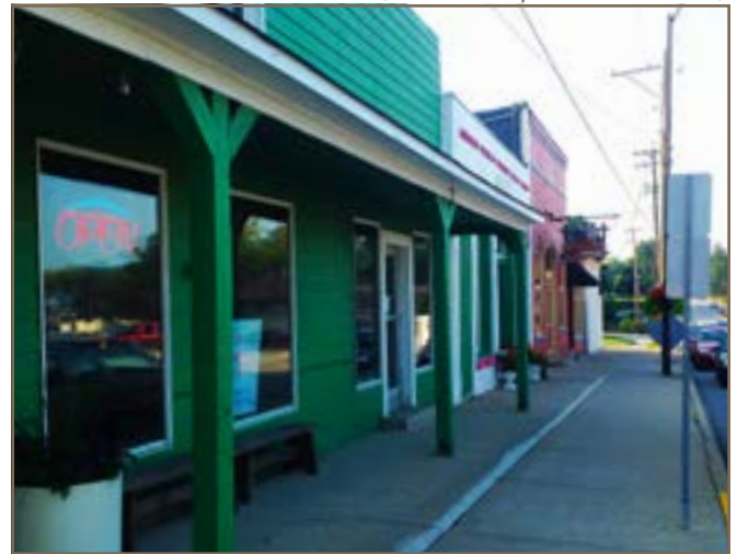
Figure 2.8: Existing Union Street Buildings (Source: Department Photo)
