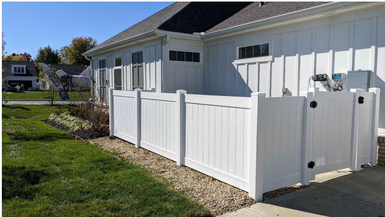
HVAC/POOL EQUIPMENT ENCLOSURE (TYP.)
