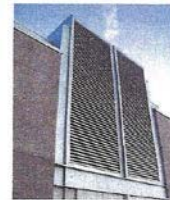
ARCHITECTURALLY LIT LOUVER PANELS
