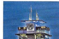
ARCHITECTURAL LIT TOWERS
