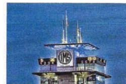
ARCHITECTURAL LIT TOWERS
