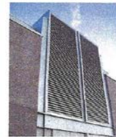
ARCHITECTURALLY LIT LOUVER PANELS
