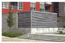
LOUVERED MECHANICAL SCREENS
