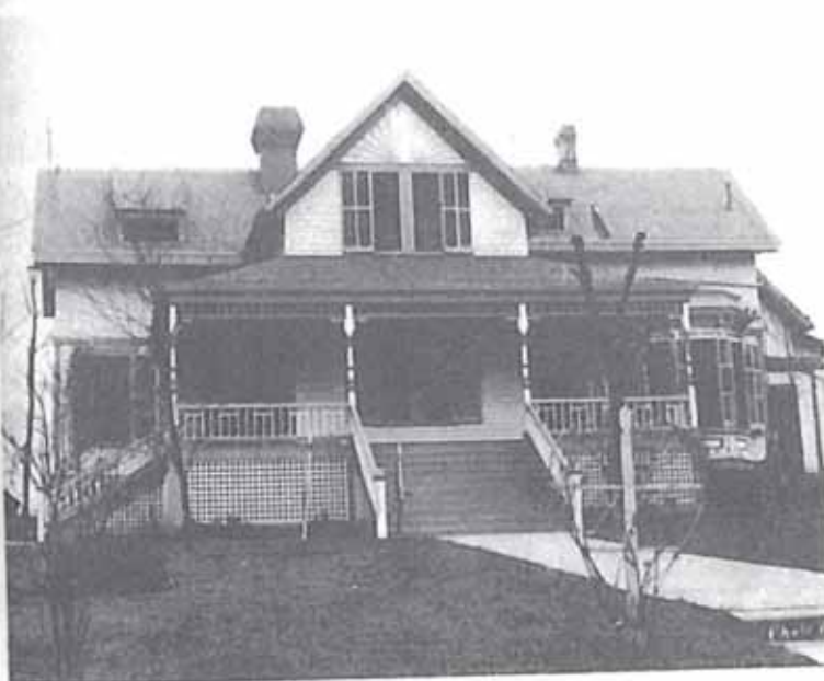
Figure 505 – Side-gabled Roof, One-Story Folk Victorian Examples
