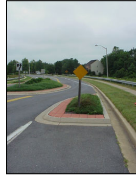
Figure 8: A traffic-calming device.
