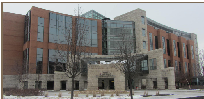
Figure 4.3 (Photo Source: Department Photo)
