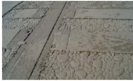
Stamped Concrete Paths & Textured Pedestrian Crossings
