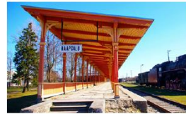
Covered Porches and Walkways
