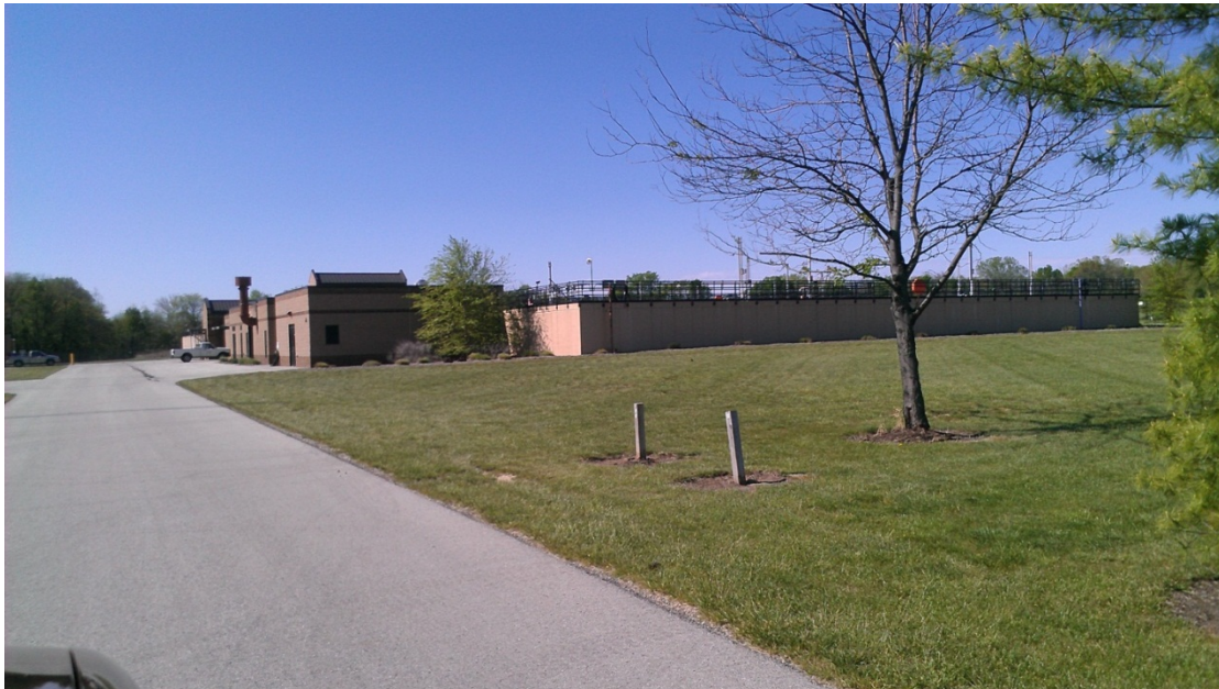
The WWTP is located on a large site with plant expansion potential
