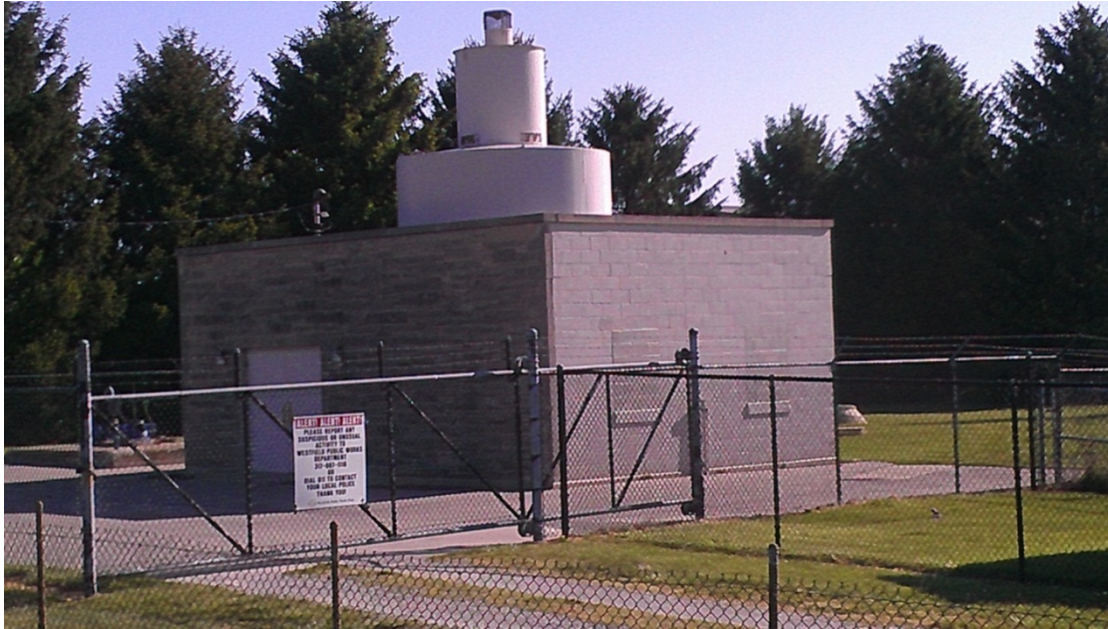
The North Wellfield and Treatment Plant are currently used as backup supply
