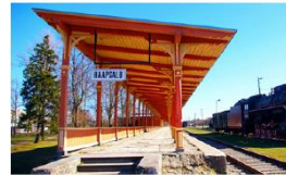
Covered Porches and Walkways
