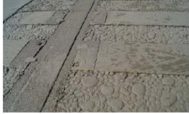
Stamped Concrete Paths & Textured Pedestrian Crossings
