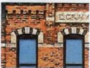
Prominent Masonry Patterns, accents, and textures. Stone Sills & Lintels in Brick Walls, Etc.
