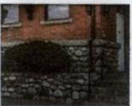
Masonry Water Table/Base Detail
