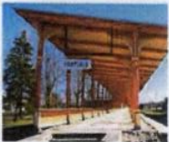
Columns with an Articulated Base, Middle, and Top.
