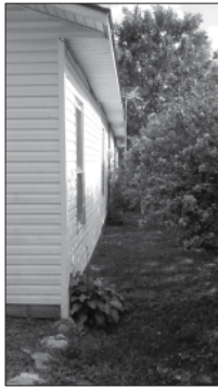
EXISTING VIEW OF NORTHWEST CORNER LOOKING SOUTH (LEFT)
