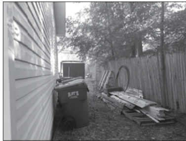
EXISTING VIEW OF SOUTHEAST GARAGE LOOKING NORTH
