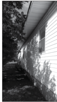
EXISTING VIEW OF SOUTHWEST CORNER LOOKING NORTH (LEFT)
