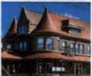
Roof Elements - Dormers, Turrets, Cupolas, Chimneys, etc.
