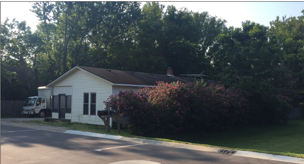
VIEW FROM PARK STREET (NORTH WEST)
