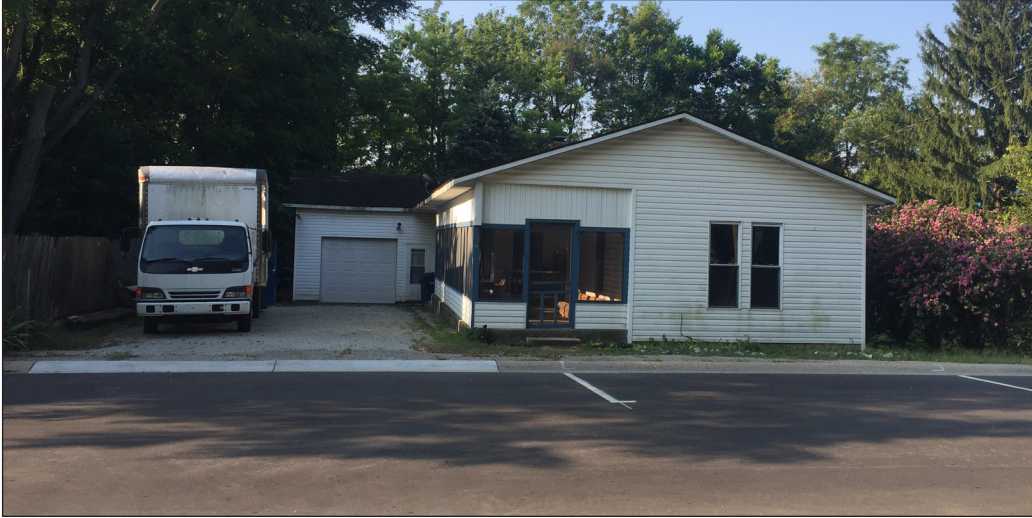
VIEW FROM REAR YARD (SOUTH)
