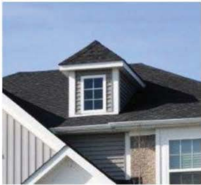
c. Dutch hip (Gable over hip roof)
