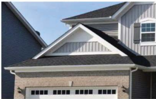
d. Jerkinhead (Hip over gable roof)
