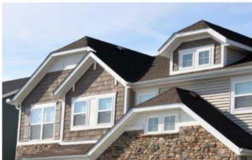
d. Jerkinhead (Hip over gable roof)
