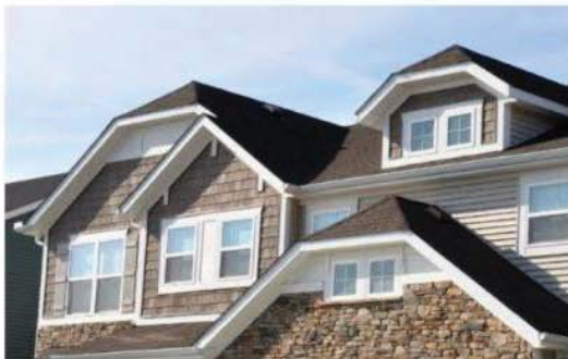
d. Jerkinhead (Hip over gable roof)
