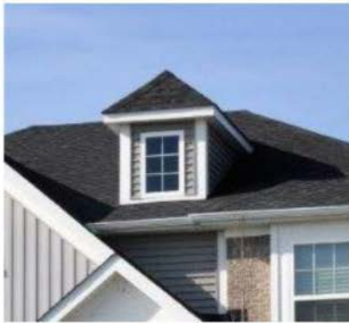
c. Dutch hip (Gable over hip roof)
