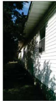
EXISTING VIEW OF SOUTHWEST CORNER LOOKING NORTH (LEFT)
