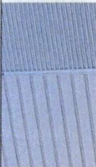
Metal Panel Siding
