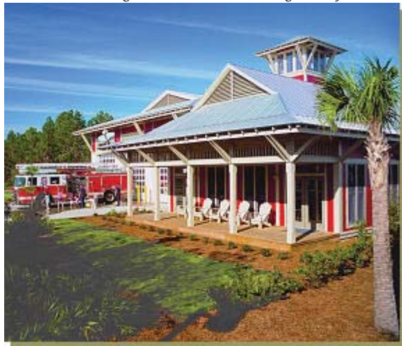
Figure 12 Hardie Plank siding variation with New England style architecture
