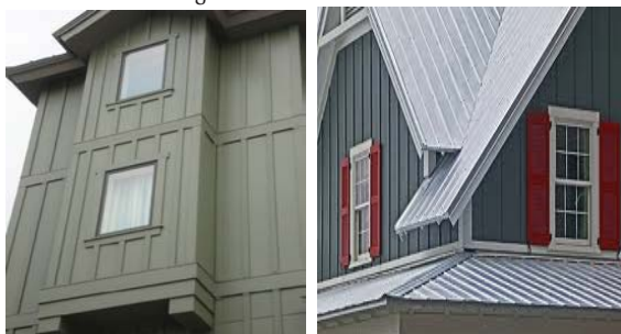
Figure 13 Hardie Plank siding variations
