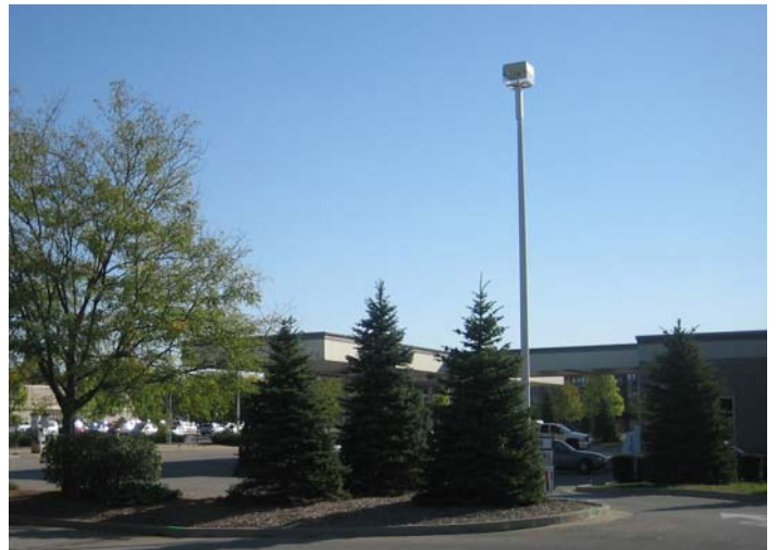
Example 6 – Fuel Station
