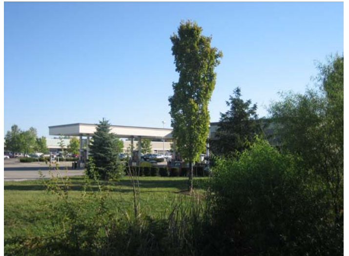
Example 4 – Fuel Station
