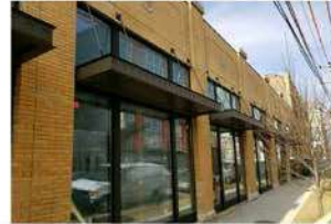
BRICK VENEER/METAL CANOPIES
