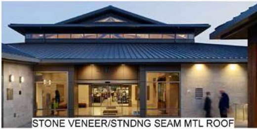
STONE VENEER/STNDNG SEAM MTL ROOF
