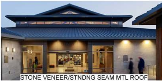
STONE VENEER/STNDNG SEAM MTL ROOF
