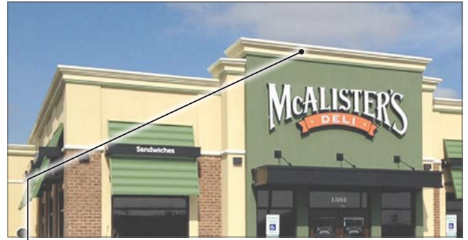
articulated three-dimensional cornice
