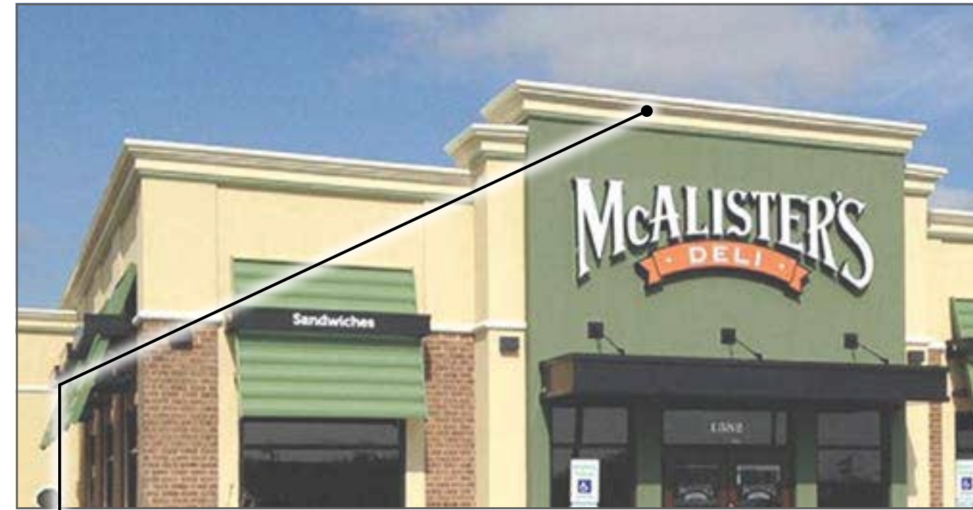
articulated three-dimensional cornice
