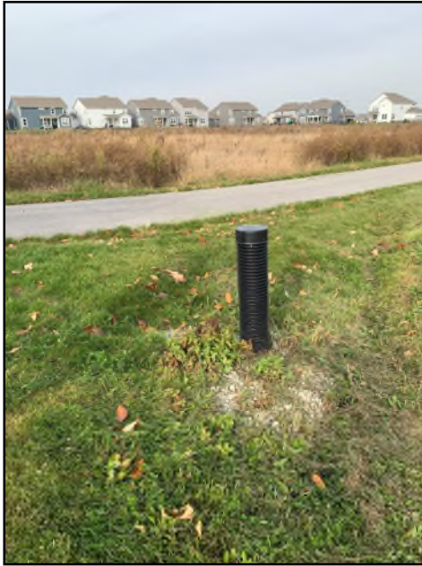
Drainage inlet on west side of property
