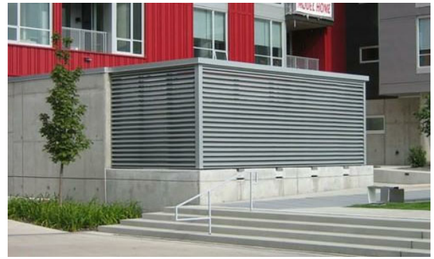
LOUVERED MECHANICAL SCREENS
