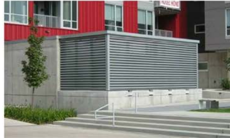
LOUVERED MECHANICAL SCREENS
