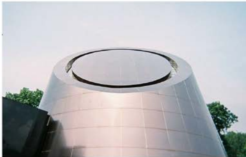
METAL PANEL ROOFS AND FACADE
