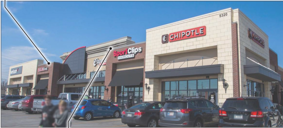
roof line modulation
