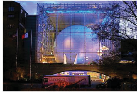
GLASS STOREFRONT TO EXPOSE INTERIOR PLANETARIUM DOME
