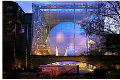
GLASS STOREFRONT TO EXPOSE INTERIOR PLANETARIUM DOME
