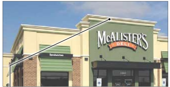
articulated three-dimensional cornice
