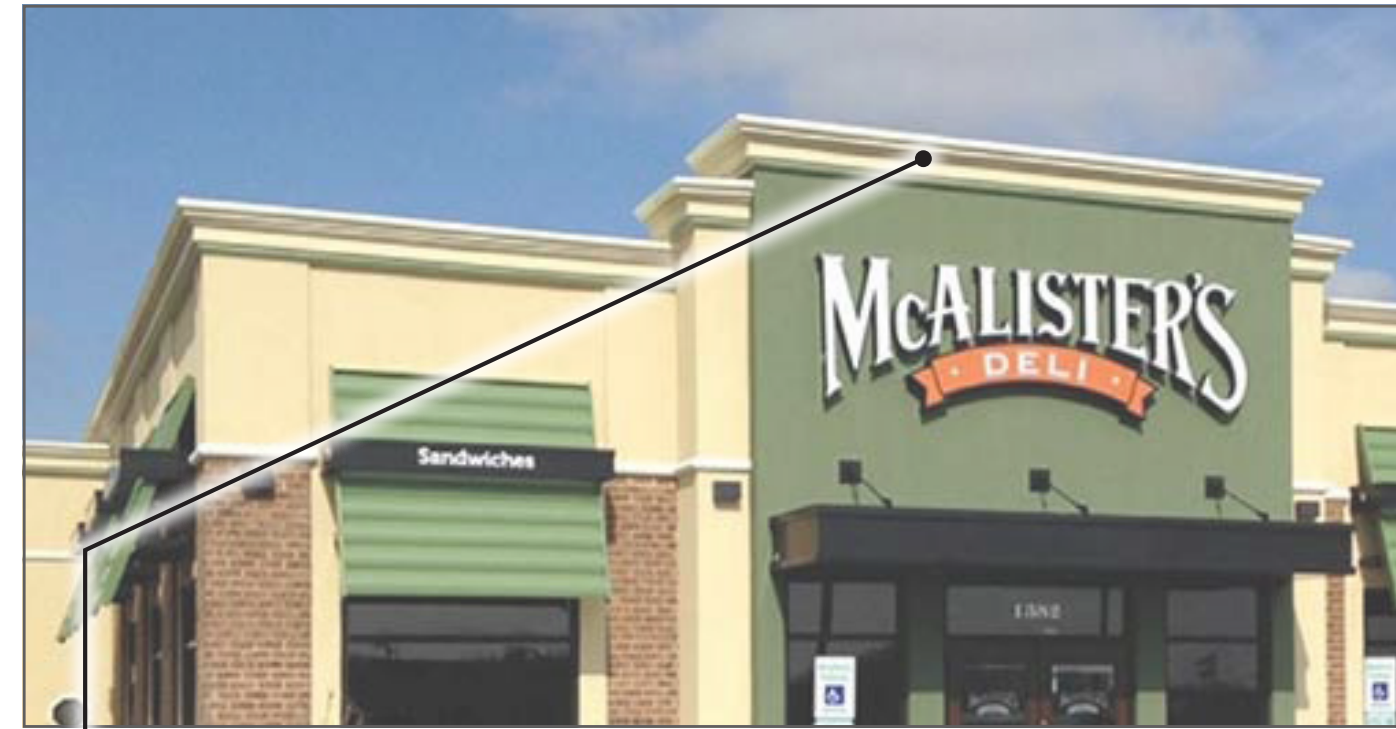
articulated three-dimensional cornice
