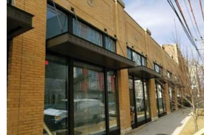
BRICK VENEER/METAL CANOPIES
