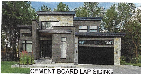
STONE VENEER/STNDNG SEAM MTL ROOF
