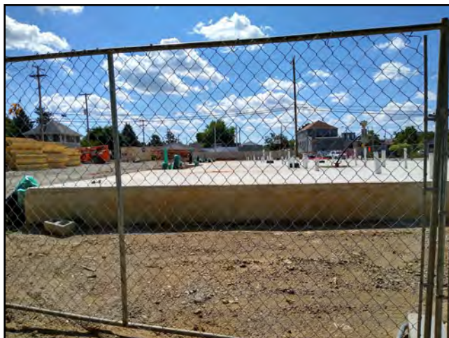
Photo View Looking south
