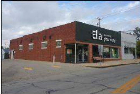
Photo View Looking NW from Union St.
