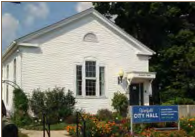
Figure 2.14: Existing City Hall (Source: Department Photo)
