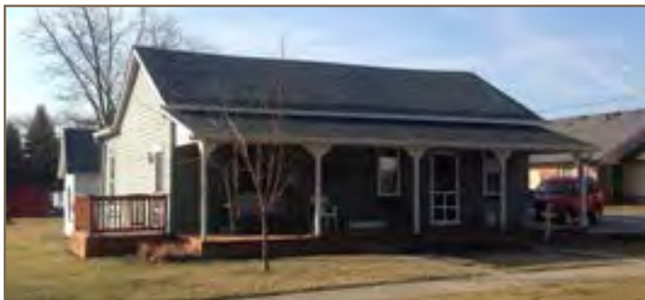
(10) Oscar Brown House (Contributing), 136 N Union Street. Italianate, c. 1879; Architecture (Interim Report No. 018).
