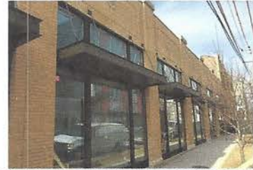
BRICK VENEER/METAL CANOPIES
