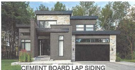
CEMENT BOARD LAP SIDING
