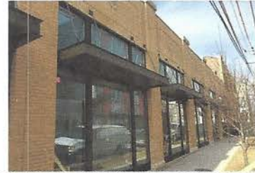
BRICK VENEER/METAL CANOPIES
