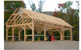
HEAVY TIMBER STRUCTURE
