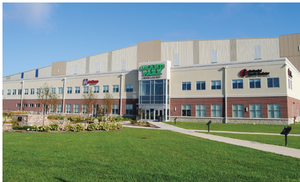
Figure 3.2: Grand Park Event Center (above) is a 377,000 square feet indoor recreation facility located at 19000 Grand Park Boulevard, Westfield, IN 46074.
