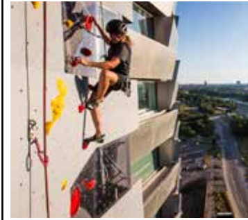
Climbing Wall Facade
