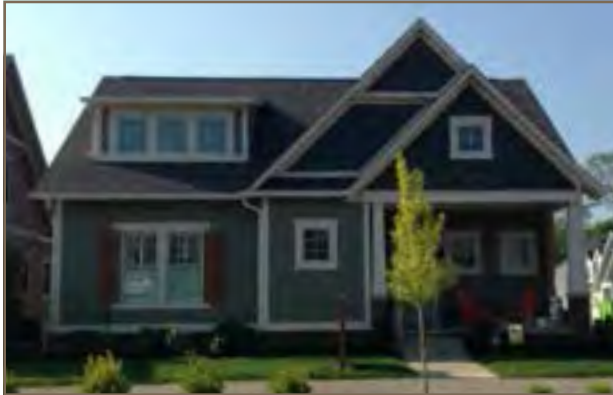
Figure 2.13.D (Source: Department Photo)
