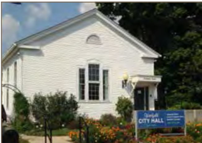
Figure 2.14: Existing City Hall (Source: Department Photo)
