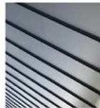
STANDING SEAM METAL SIDING AND ROOF
