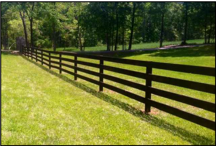
ILLUSTRATION - TYPICAL FOUR-BOARD HORSE FENCING
