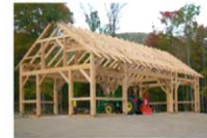
HEAVY TIMBER STRUCTURE
