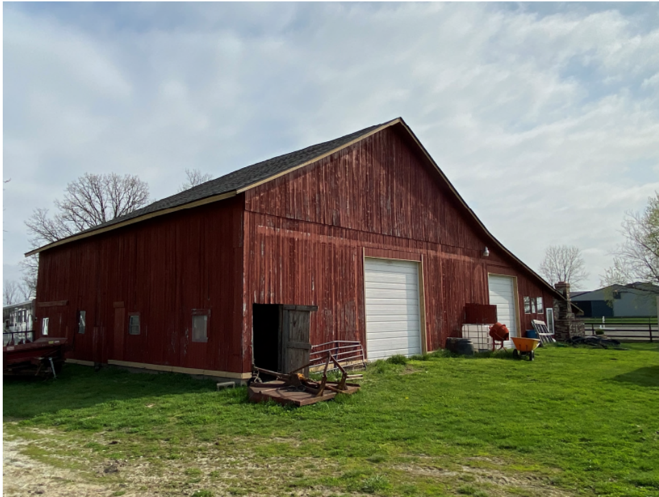
South side of Cidery Building
