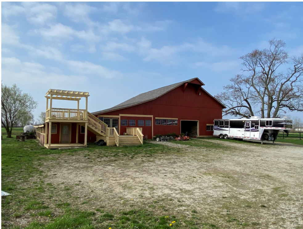
North side of Cidery Building
