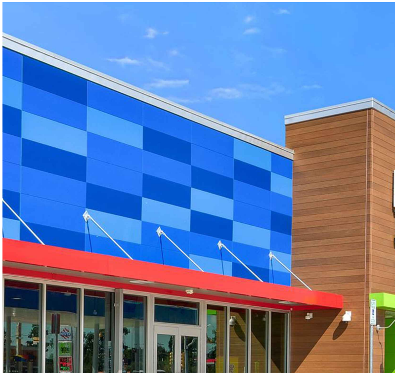
NICHIHA ARCHITECTURAL WALL PANELS (TYP) ILLUMINATION SERIES
