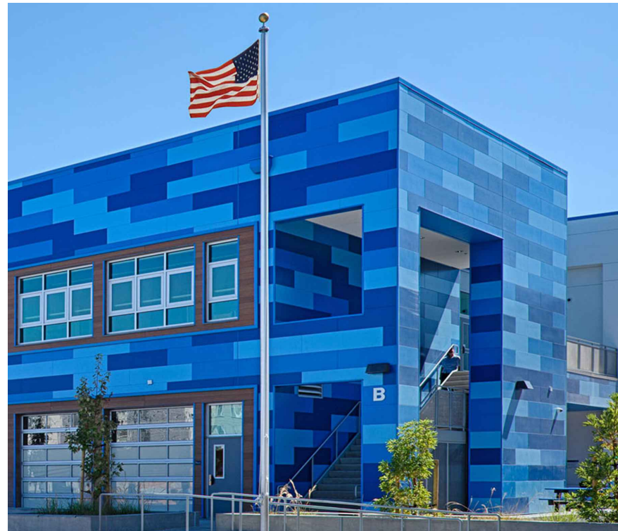
NICHIHA ARCHITECTURAL WALL PANELS (TYP) ILLUMINATION SERIES
