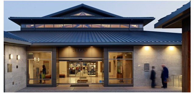
STONE VENEER/STANDING SEAM METAL ROOFING
