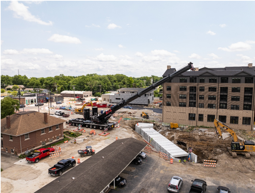
14' x 6' Box Culvert Install
