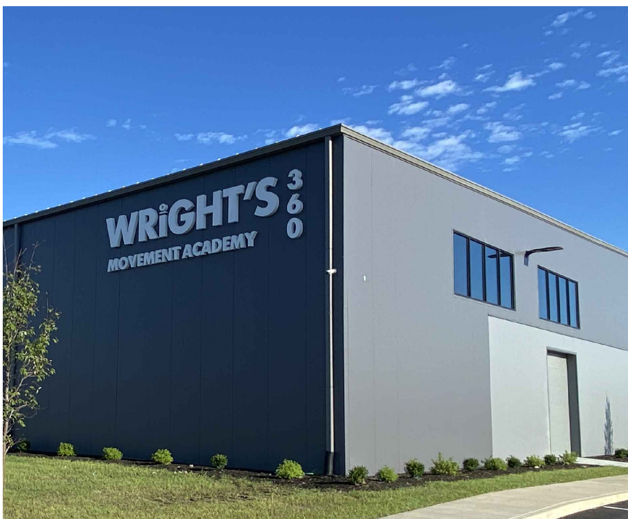
VERTICAL METAL SIDING WRIGHT'S MOVEMENT ACADEMY WESTFIELD, INDIANA
