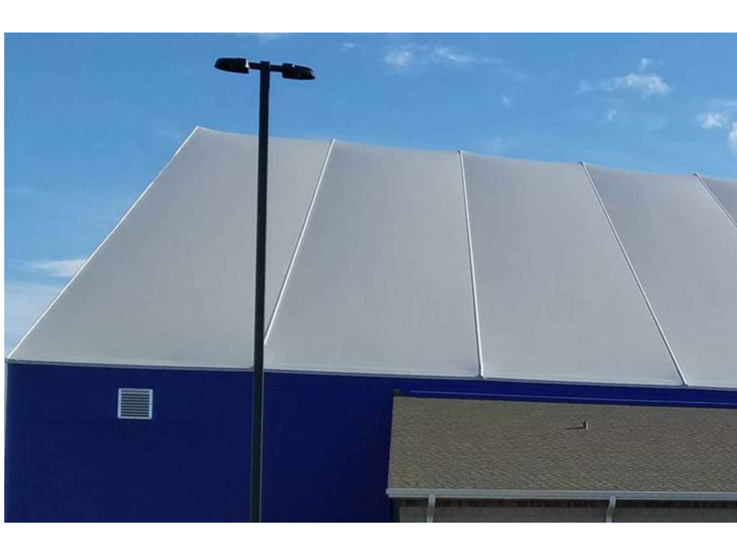
SHELTER-RITE ARCHITECTURAL FABRIC ROOF
