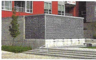
LOUVERED MECHANICAL SCREENS
