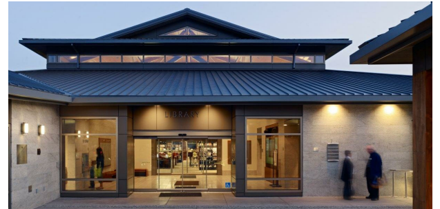
STONE VENEER/STANDING SEAM METAL ROOFING
