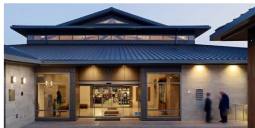
STONE VENEER/STANDING SEAM METAL ROOFING
