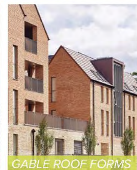
GABLE ROOF FORMS
